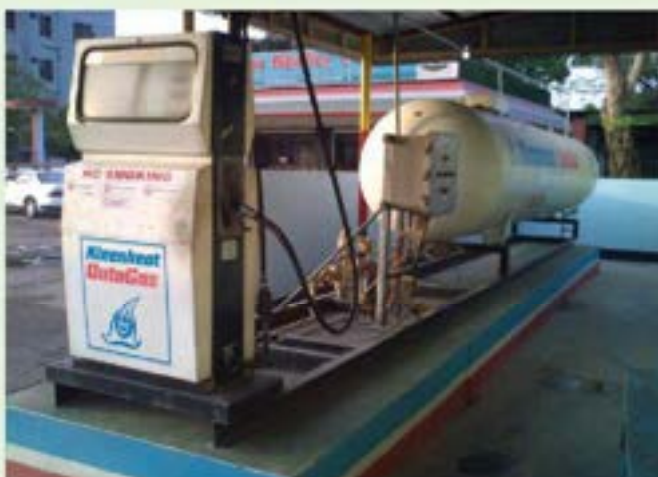
Figure 1: An autogas site at Jessore
